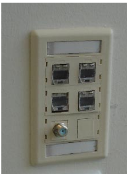
Four XG shielded copper ports plus one coax port fit in a single gang outlet.
